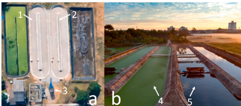
Fig. 2. a) Ponds before the start of the operation (1) Microalgae pond; (2) Macrophyte pond; (3) UASB reactor and b) Ponds after the start of the operation: (4) Microalgae pond and (5) Macrophyte pond.
