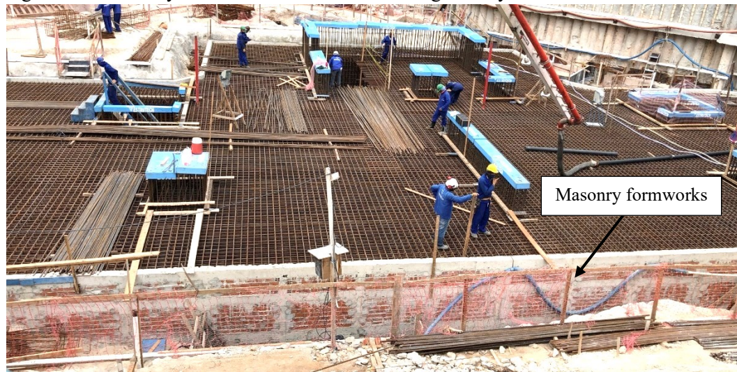
Figure 62 – Masonry formworks on the sides of the geometry
