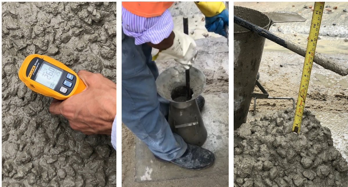
a) Measuring concrete placing temperature
