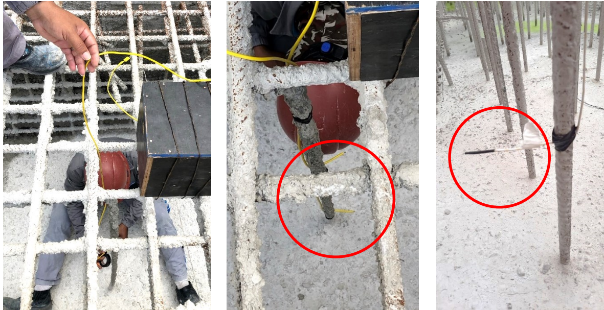
Figure 73 – Installation of thermocouples on the raft foundation reinforcement
