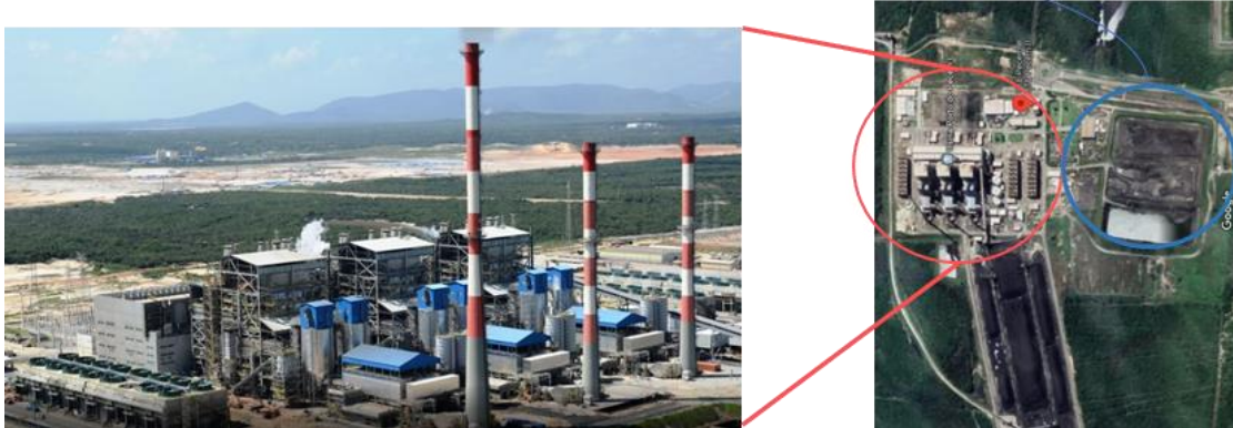
Figure 2.12 - Thermoelectric Complex Production of Pecém
