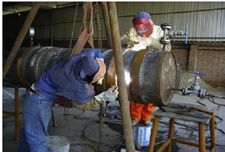
Figure 1.1 – In-service welding technique.
