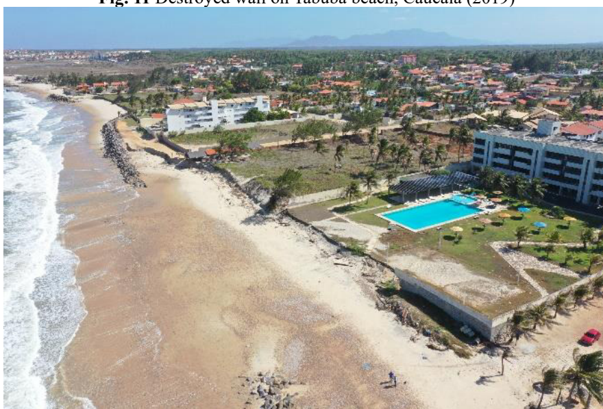
Fig. 11 Destroyed wall on Tabuba beach, Caucaia (2019)
