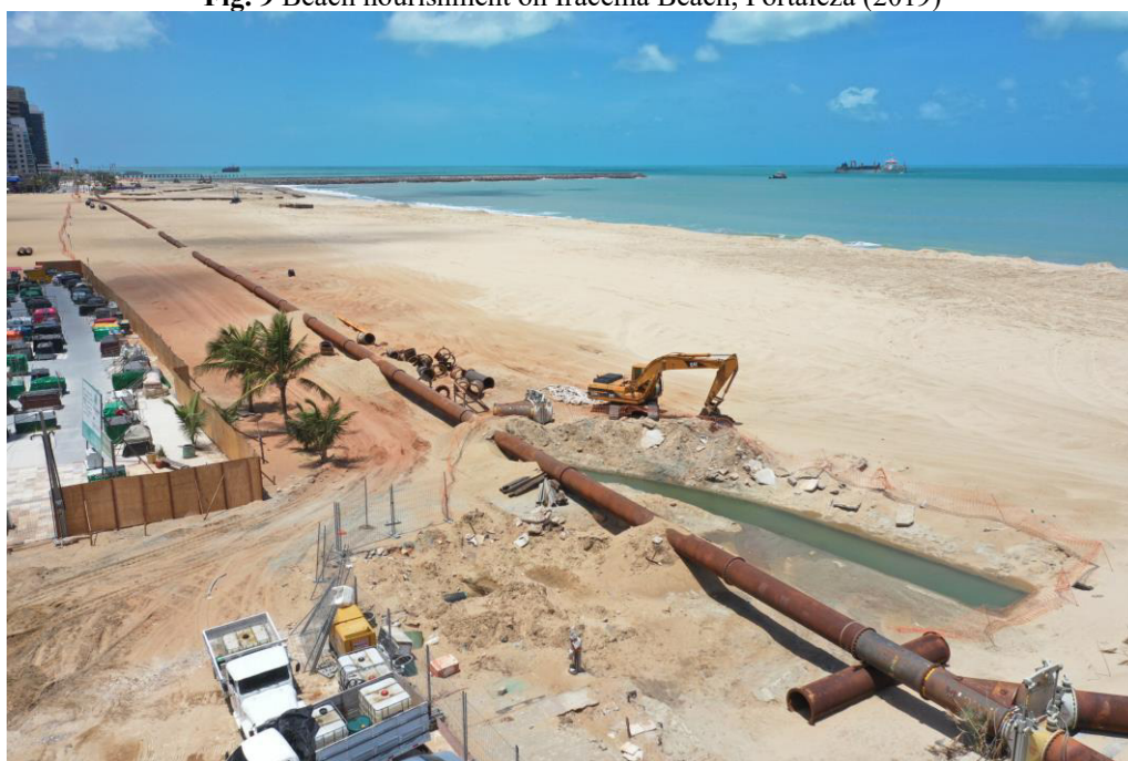
Fig. 9 Beach nourishment on Iracema Beach, Fortaleza (2019)
