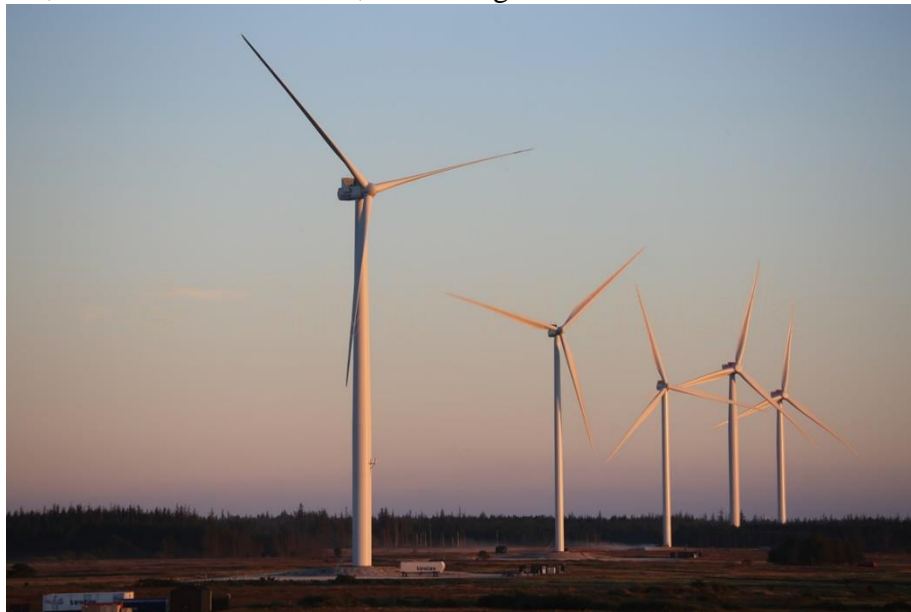
Figure 3 – Horizontal-axis wind turbine: Vestas V126, rated power 3.45 MW, rotor diameter 126.0 m, tower height 137 m
