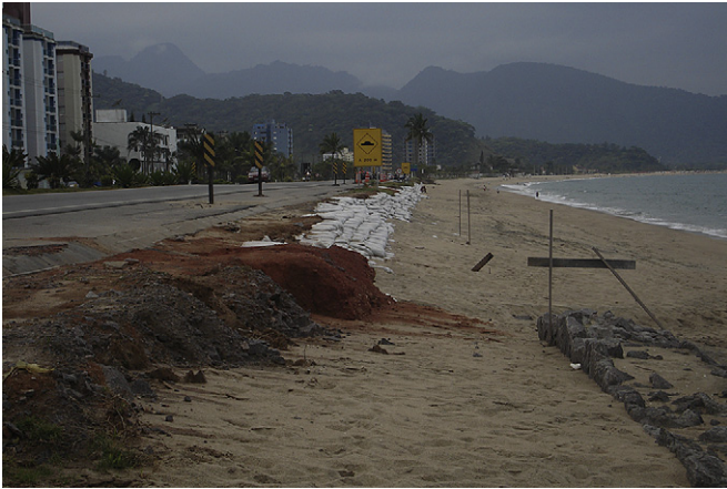
Fig. 6. Coastal engineering structures in Sector 2 (2006).
