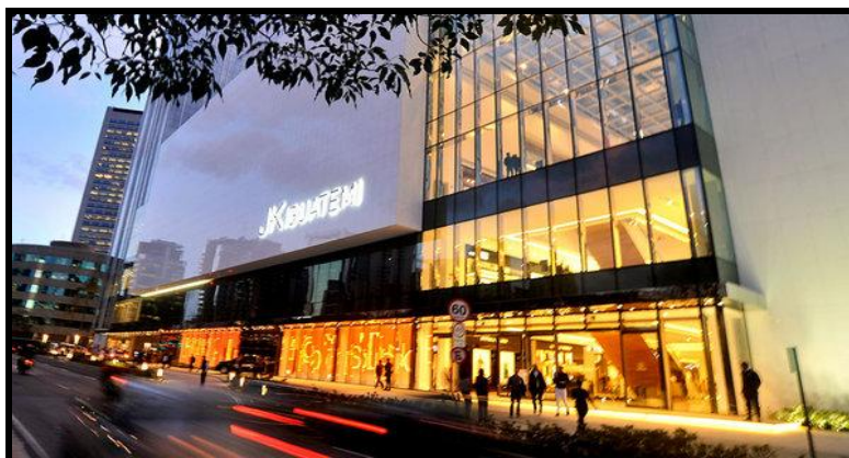
Figura 3 – Fachada do Shopping JK Iguatemi
