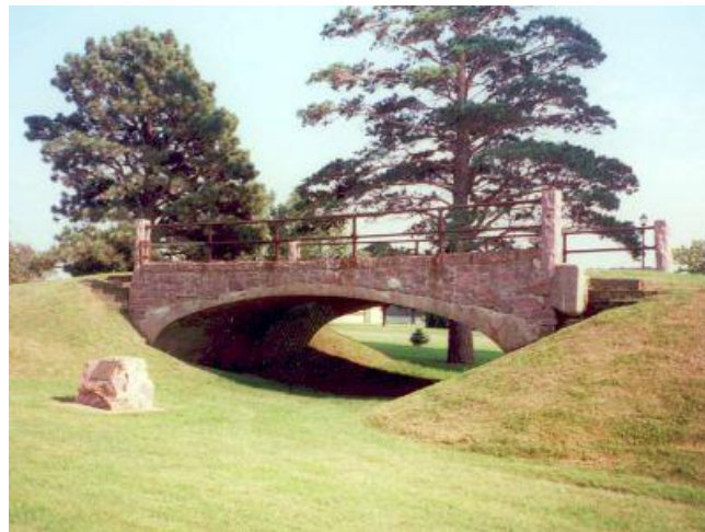
Figura 1 - Ponte Rock Rapids Bridge , Iowa, E.U.A.
