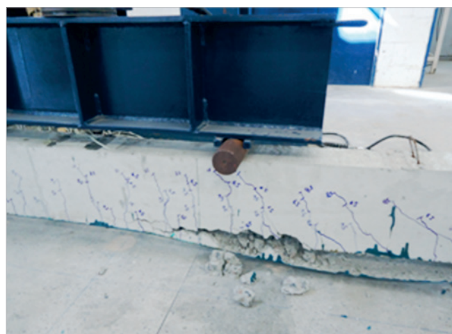
E VB-5 beam in the collapse
