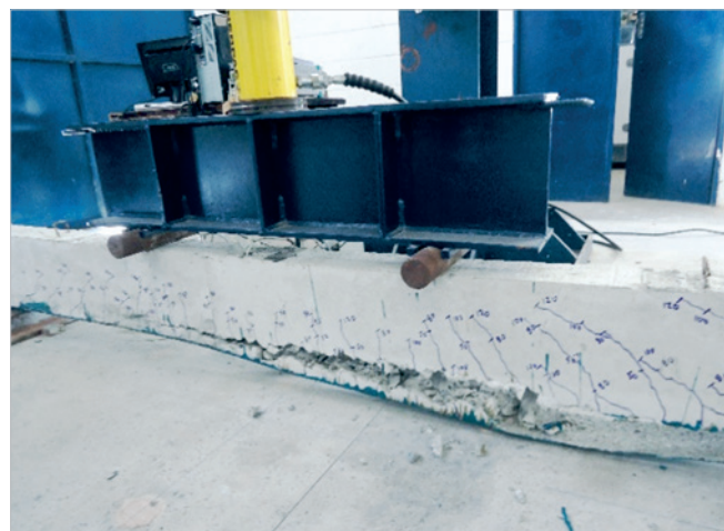
E VA-5 beam in the collapse
