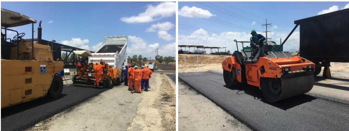
(a) asphalt paver and pneumatic roller
