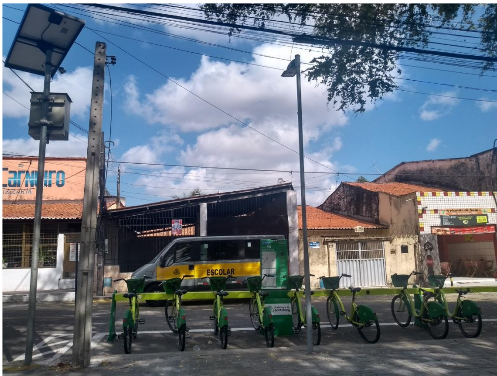
The solar panel is in the foreground / Station is balanced
