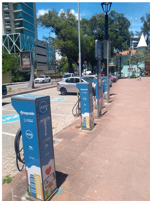
Station totem, with instructions for use / Four exclusive parking spaces and charging points installed on the square
