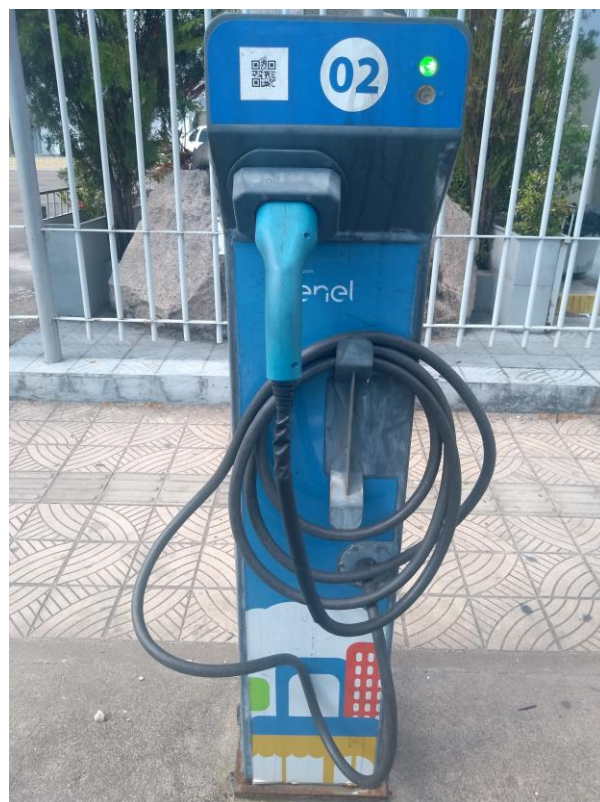
Station totem, with instructions for use / A charging point in detail (the QR code is used when returning a car to the station)
