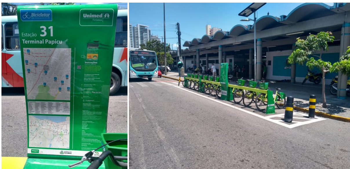
Station's totem / View of the station installed on the street, in front of the bus terminal (station is imbalanced)
