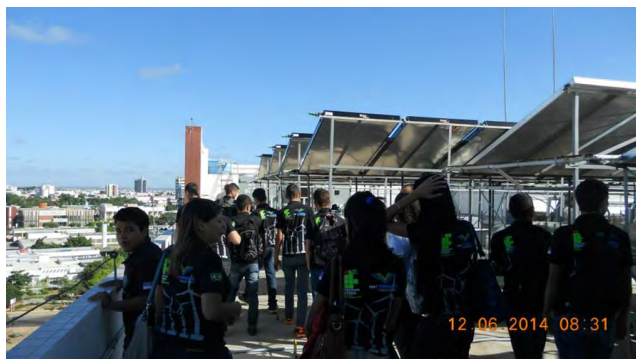
FIGURE 7. Solar heating systems visit in petrolina-pernambuco-brazil.
