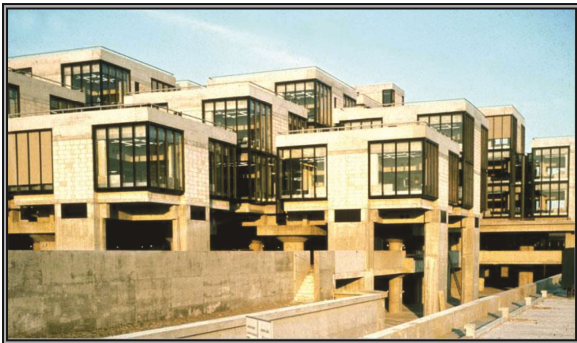
Fig. 6. Central Beheer Offices Apeldoorn
