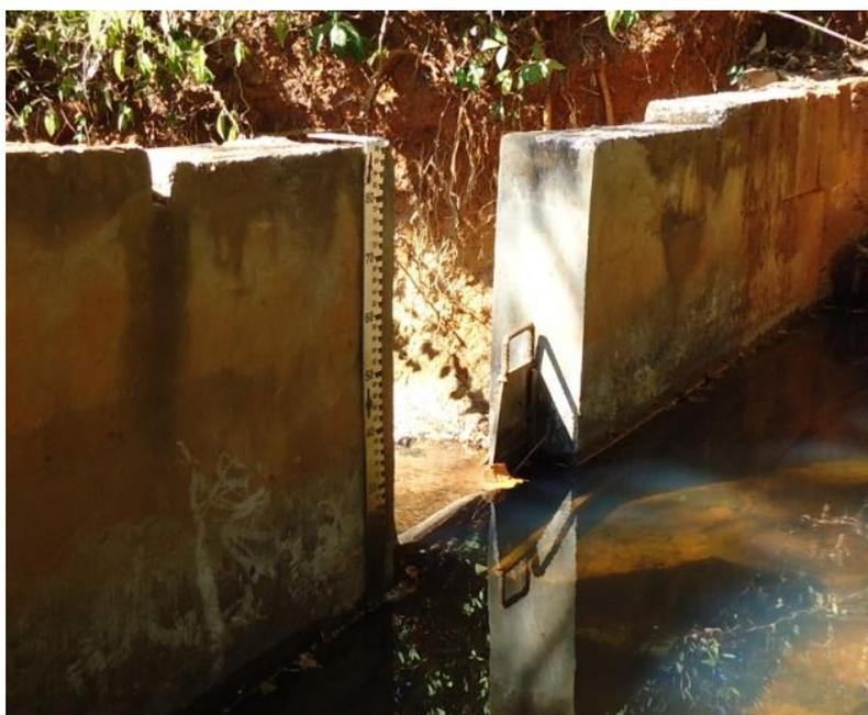
**Figura 4.4 - Vertedouro trapezoidal de base 40cm (VTMA01) – Abr/2010**
