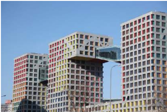
Imagem 31: Fachada multicolorida Fonte: https://www.archdaily.com/34302/linked-hybrid-steven-holl-architects
