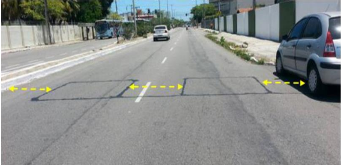
Figure 29 - Typical inductive loop-type sensor in Fortaleza street
