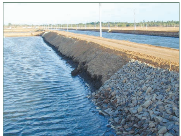
The stabilization of embankments with stone can reduce erosion and suspended solids in pond water.
