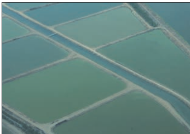
The extensive, non-aerated ponds in Latin America are typically large.
