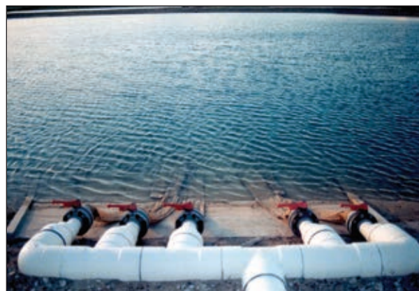
Filter bags remove vectors or pathogens from incoming water.
