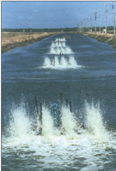
Oxidation ditch for recirculating pond water.
