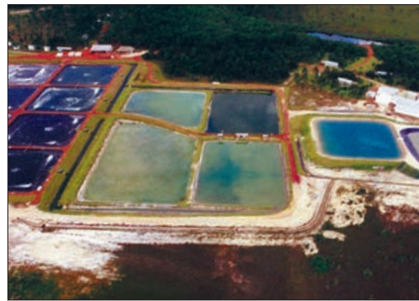
Although they represent only a small area of large farms, sedimentation basins can provide effective water treatment.
