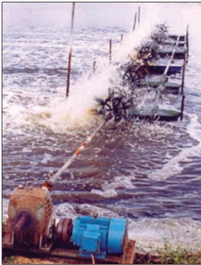
“Long-arm” paddlewheel aerators utilize multiple impellers powered by motors mounted on pond banks.
