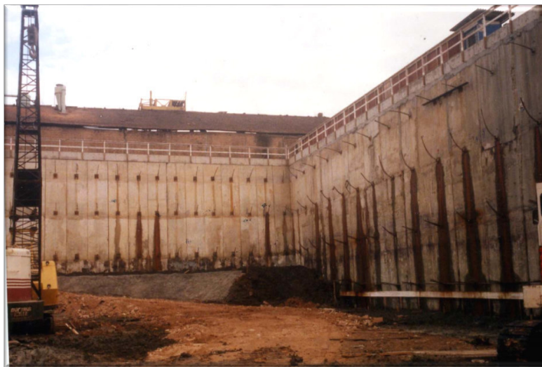
Figura 28 – Parede diafragma moldada in loco
