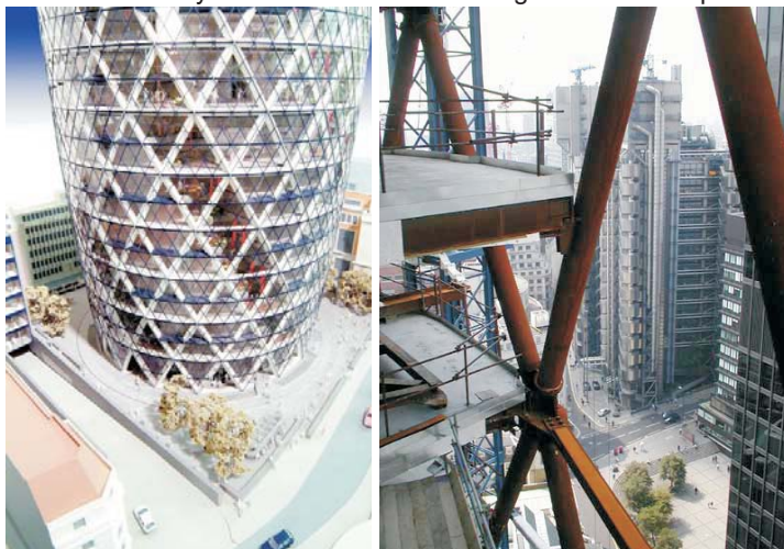
Figura 5.2.3 - Sistema estrutural Diagrid Fonte: A New System of Construction: "Diagrid Method" Explained
