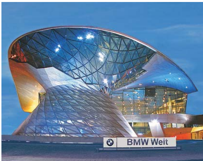
Figura 2.4.1.4 - BMW Welt - Coop Himmelbau Fonte : http://farm3.static.flickr.com/2156/2199786487_a0dd44cdd8.jpg
