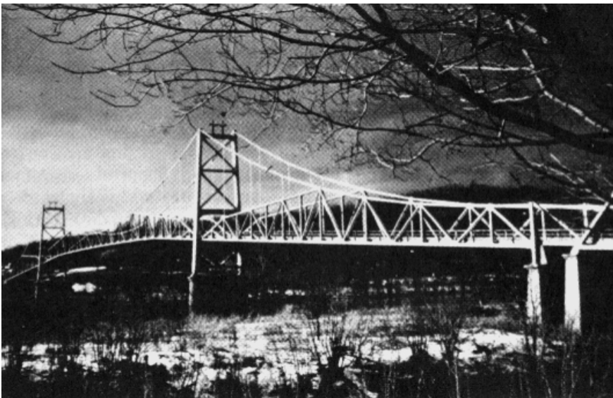
Figura 2.4 –Fotografia de St. Mary's Bridge , similar à Point Pleasant Bridge
