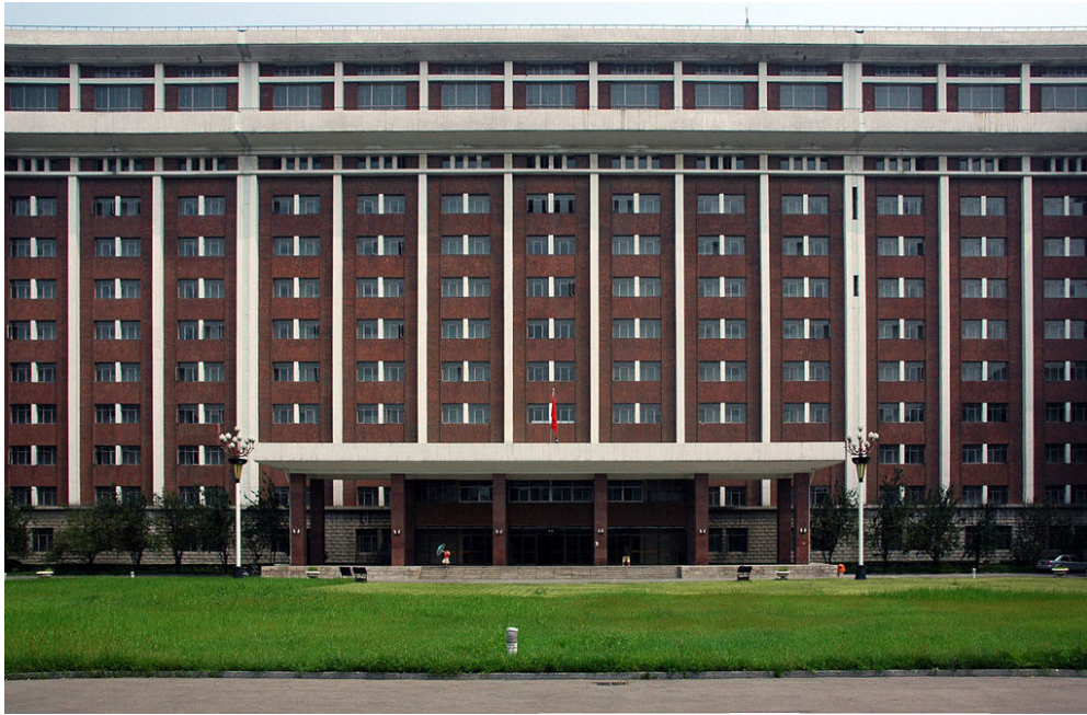
Figura 5.1: Fachada frontal de Tianjin University of Technology, Tianjin, China ( http://wikipedia.org/ ).
