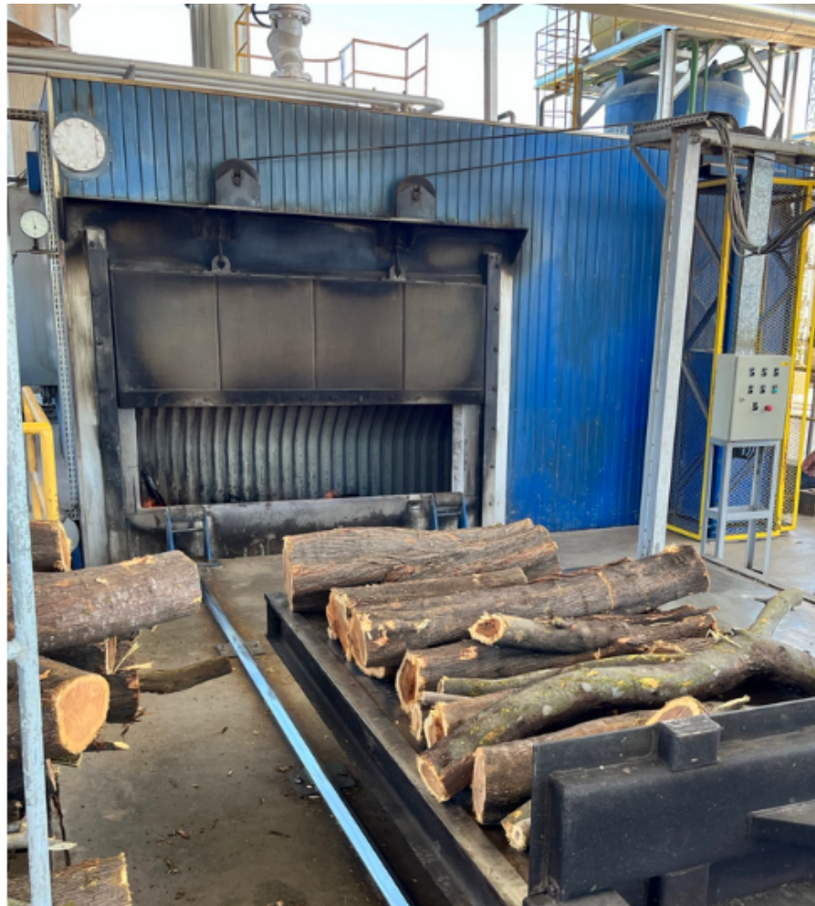
Figure 22: Ambitubular fixed grate boiler
