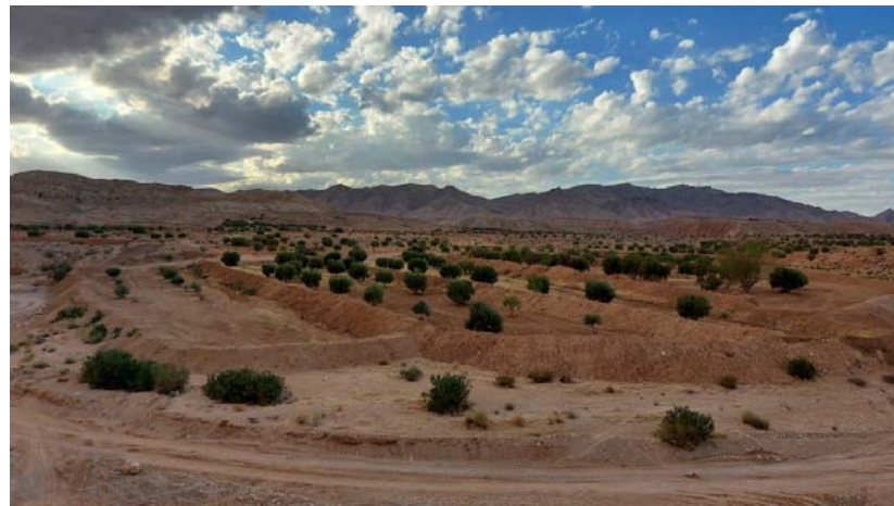
Figure 16 – Individual water erosion measure (Tabia) protection upstream in Rihana catchment in a private land
