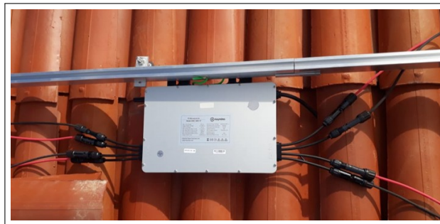
Figura 21 – Microinversor.
