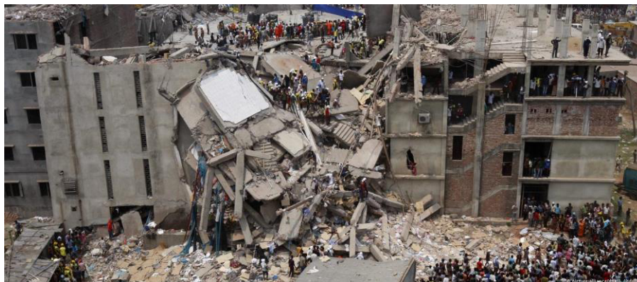
Figura 3 – Colapso Rana Plaza 2013.
