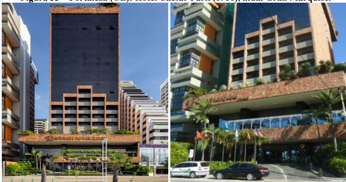
Figura 33 – Fortaleza (CE): Hotel Caesar Park (1986), atual Gran Marquise.
