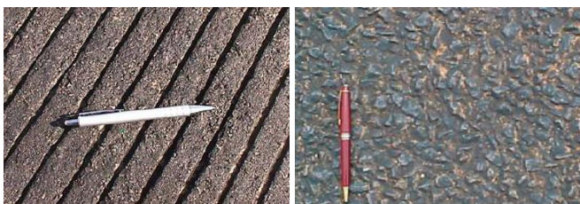
Figure 2: (a) HMA with Grooving (HMAg) e (b) Double Asphalt Surface Treatment (DAST)
