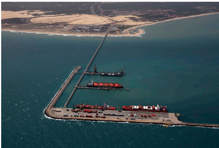
Figure 1. Aerial view of the Port of Pecém, showing the pier in 'L' and the bay of calm waters. Source: Tecer (2014).
