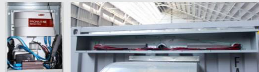
(Top) Inside a finished Anvil Crawler inverter house. (Bottom left) Pre-installed and wired Fronius weather station and monitoring. (Bottom right) Pre-wired inverter DC terminal strip.
