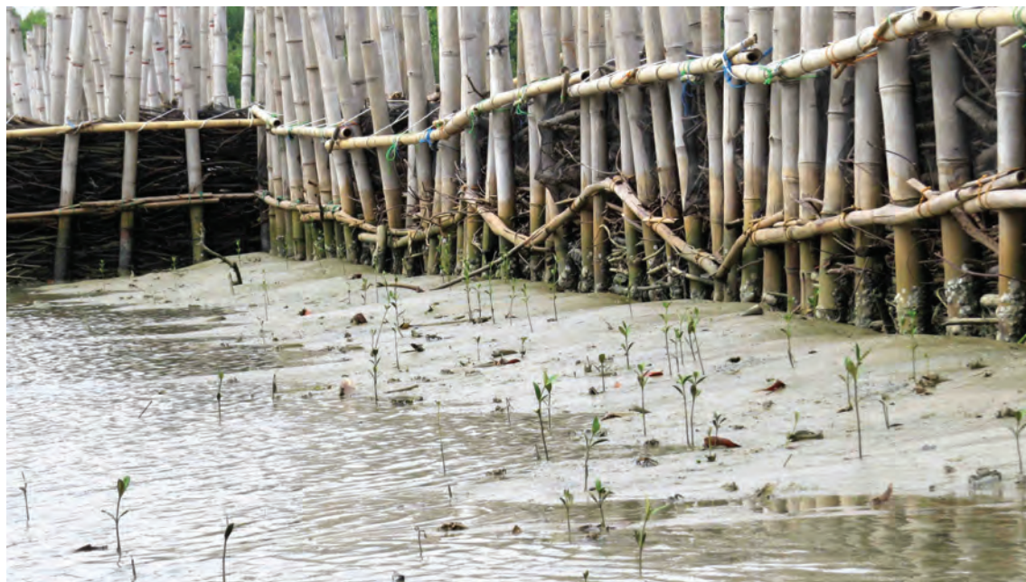
Nature's way, with help: Mangroves establish naturally behind a porous sediment trap in Indonesia. Photo: Apri Susanto
