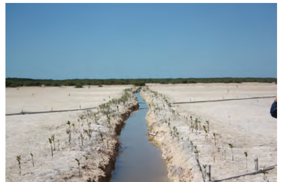
Bankable technique: The installation of canals can reduce salinity on banks and enable propagules to establish, such as these Rhizophora seedlings established by direct sowing. Photo: Jacinto Samuel García Carreón/CONAFOR
