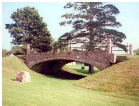
Figura 2.1 - Ponte Rock Rapids Bridge , Iowa, E.U.A.
