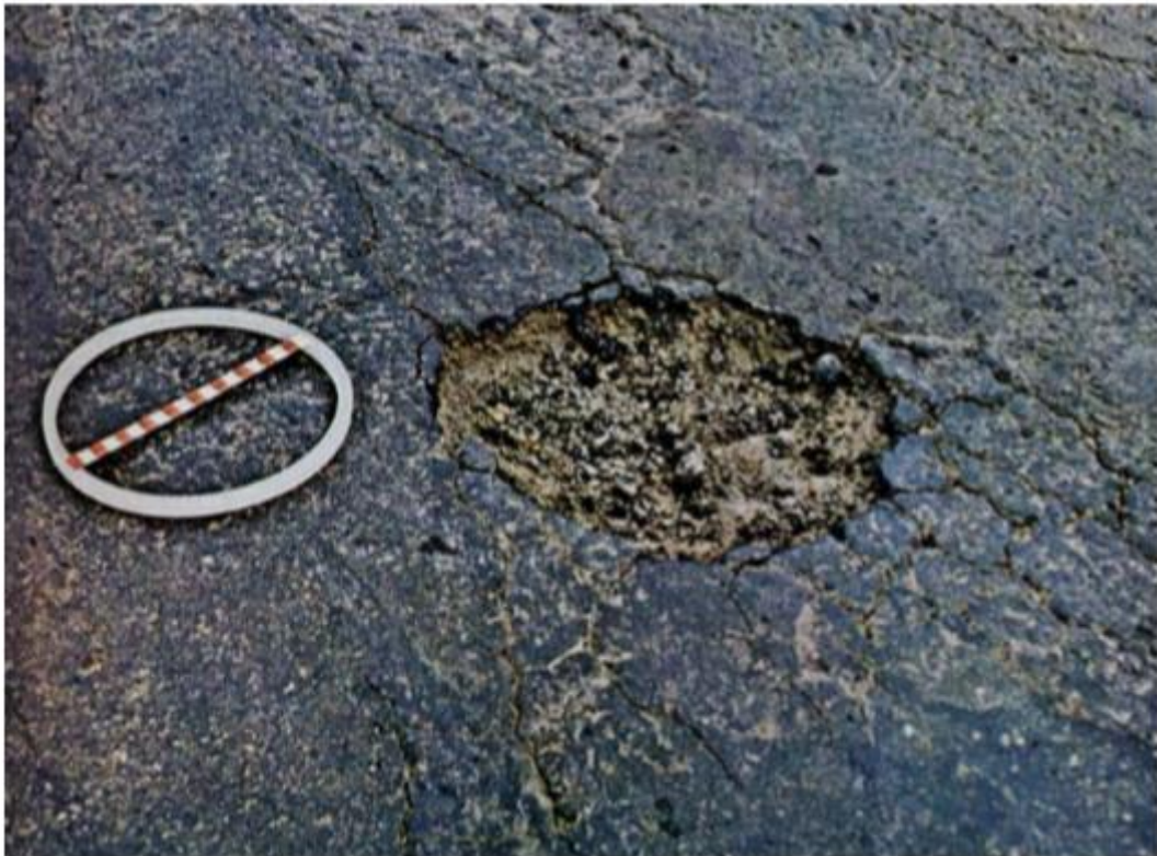
Figura 14 – Painela/buraco
