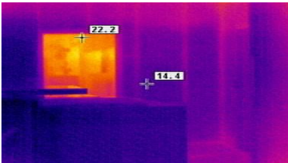
Figure 14: Temperature from the room in 2nd floor.
