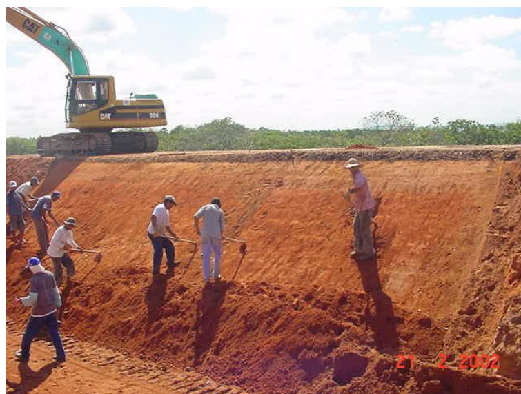
Figura 1 – Talude artificial (Talude de aterro)
